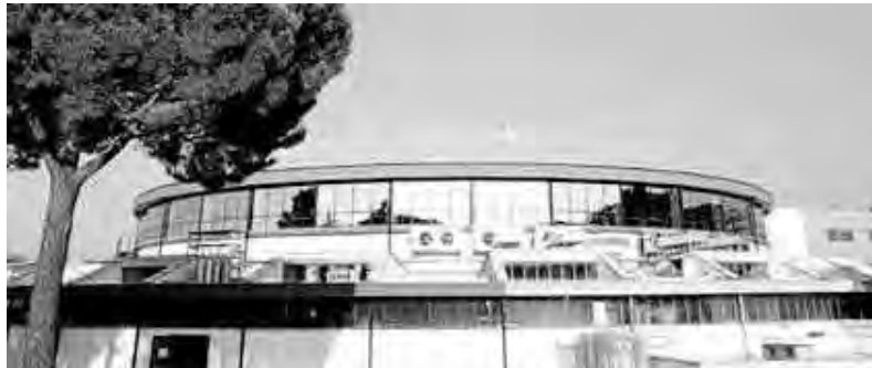
Figure 2.2: The Adone building.
